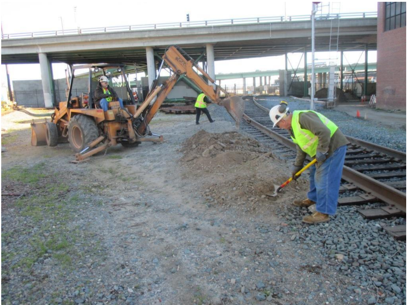
Mike F. in the back-hoe and Clem tear resurface the area to the west of the 560 Interchange Track
