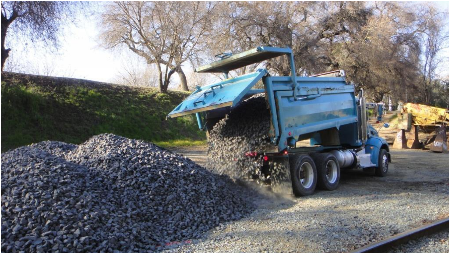
216 tons of ballast
